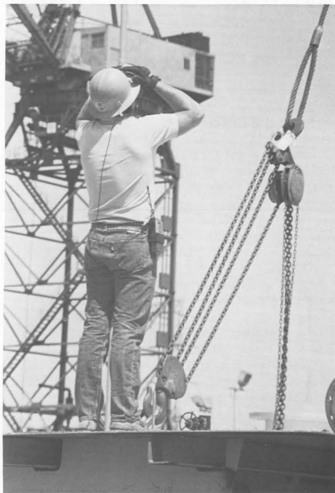
A rigger foreman supervises a typical heavy module lift. Notice the "CPR Qualified" decal on his hardhat.
